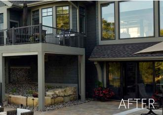
Limestone blocks were originally used under and near the deck. We re-purposed them and added a few more for the deck retaining wall (left), the wall along the conservation easement on the south side of the home, and just off the southeast corner of the pool (above).
