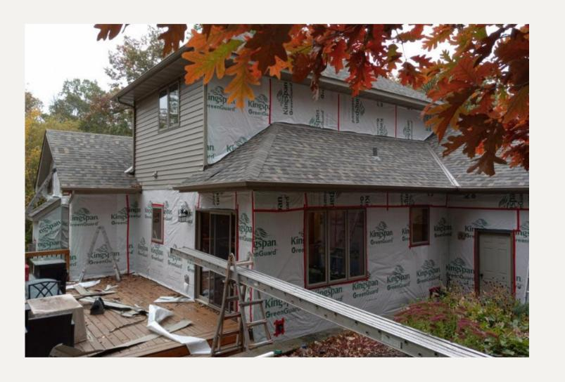
During the tear off for siding it was discovered that the soffit had been installed on top of the previous siding. This prompted us to return to insurance to get the additional soffit & fascia work covered.
