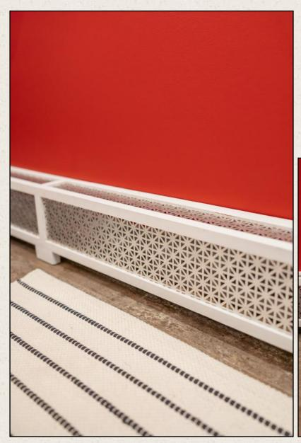
Custom-made heat cover crafted to fit over existing baseboard hot water boiler. The metal finish was coordinated with the plumbing fixtures, while the painted wood was matched to the trimwork to seamlessly integrate the element into the bathroom's design.
